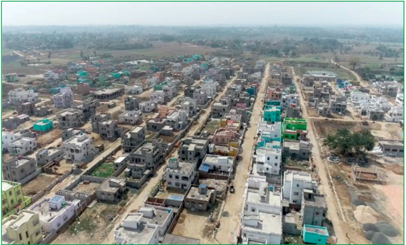
Aerial View of Rehabilitation Site of ECL
