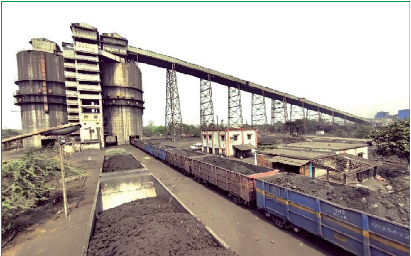
Silo Loading System at Rajmahal Area of ECL
