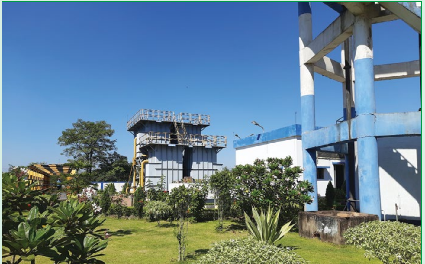
Dhandadihi Water Treatment Plant (2.0 LCuM/year)
