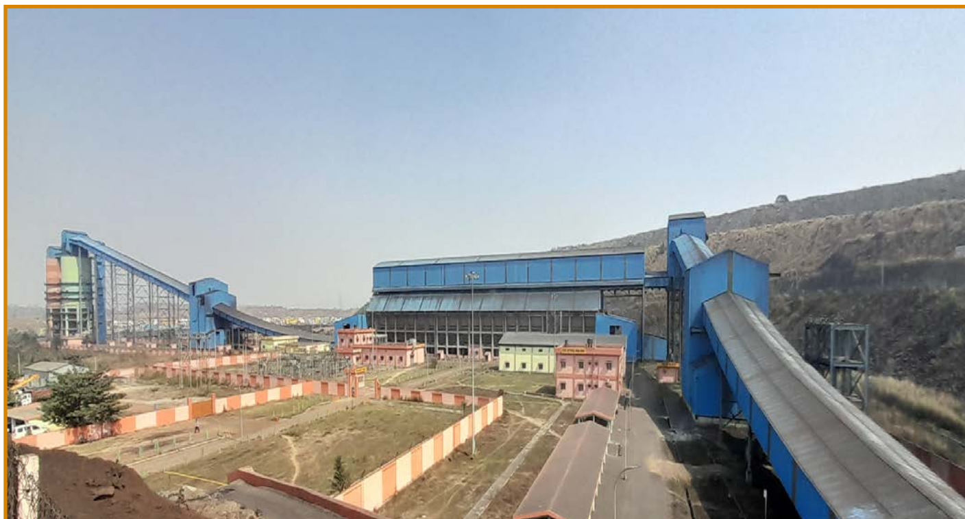
Coal Handling Plant (CHP) at Sonepur Bazari Area, ECL
