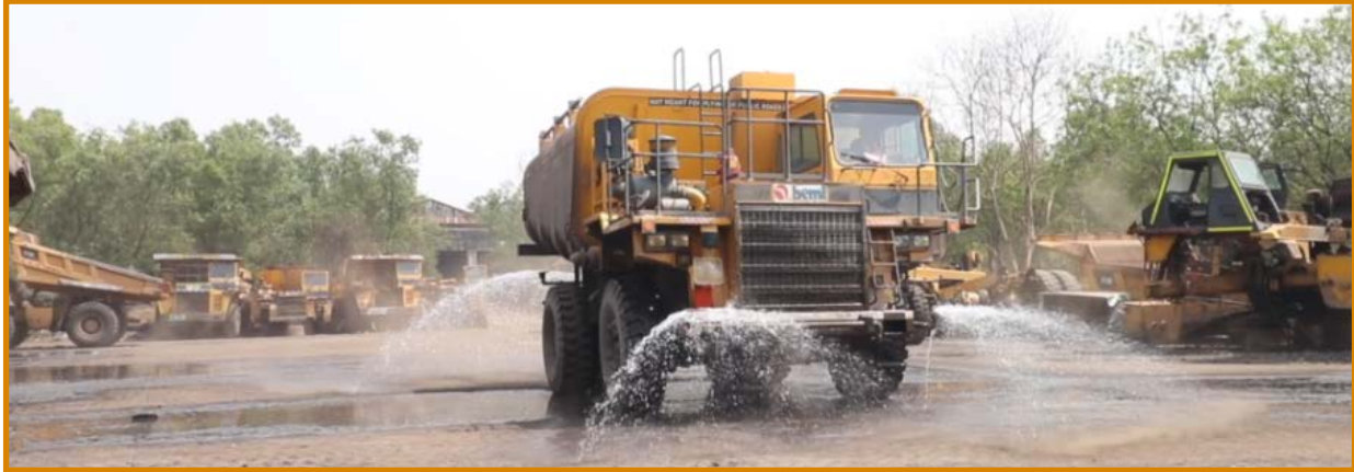
Water sprinkling for Dust suppression- A step towards sustainability
