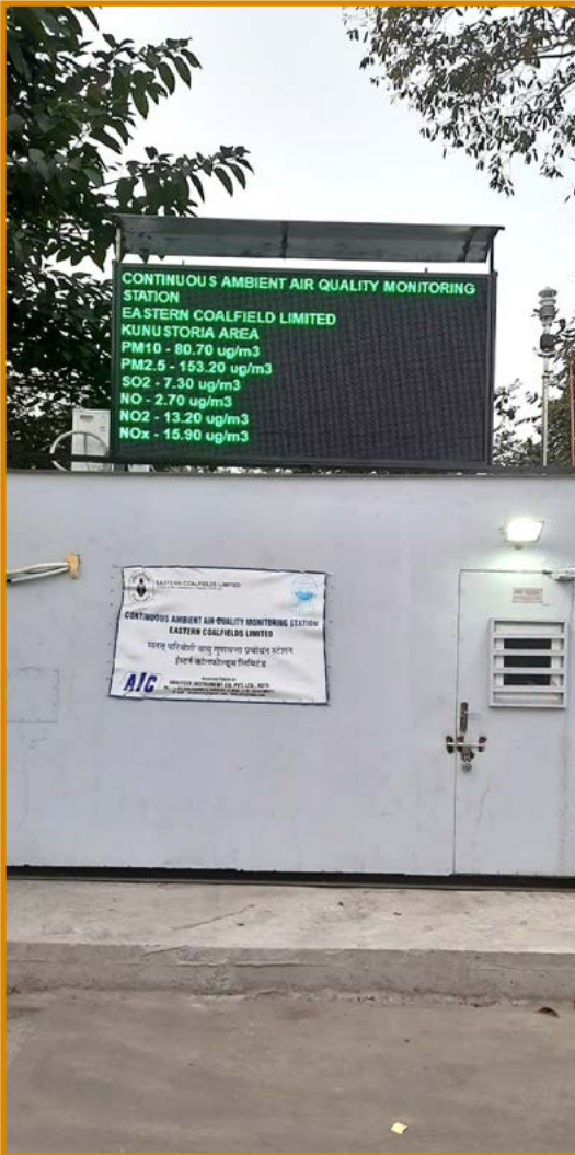
CONTINUOUS AIR QUALITY MONITORING STATION (CAAQMS) INSTALLED AT KUNUSTORIA AREA
