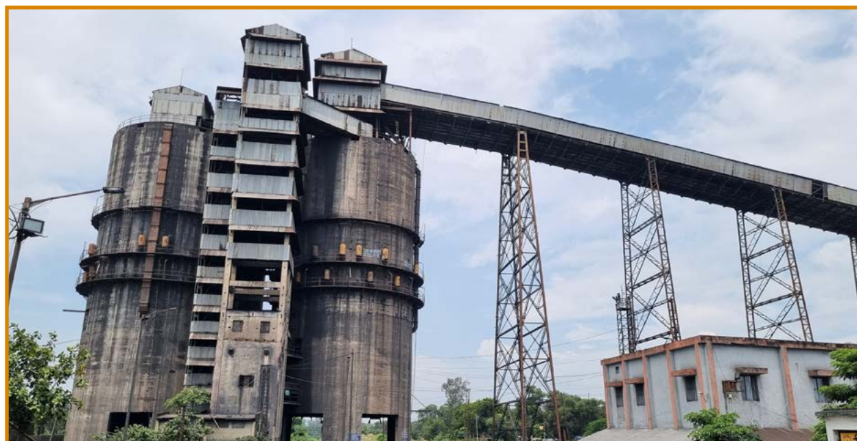
Coal Handling Plant (CHP) at Rajmahal Area of ECL
