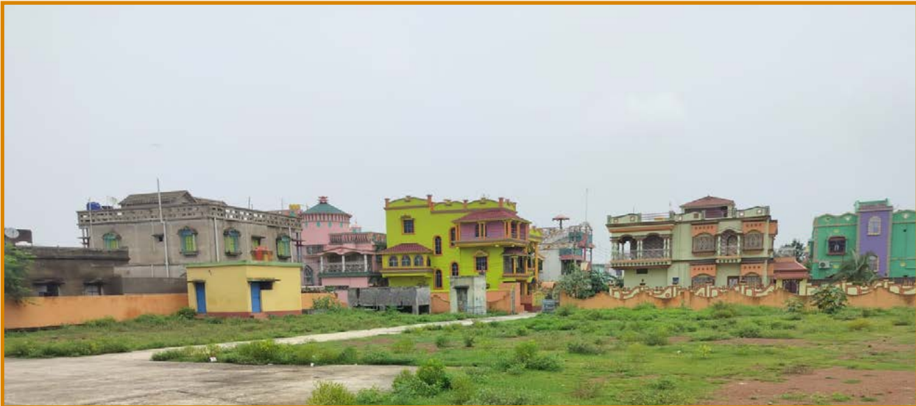
Rehab house for PAFs at Sonapur Bazari
