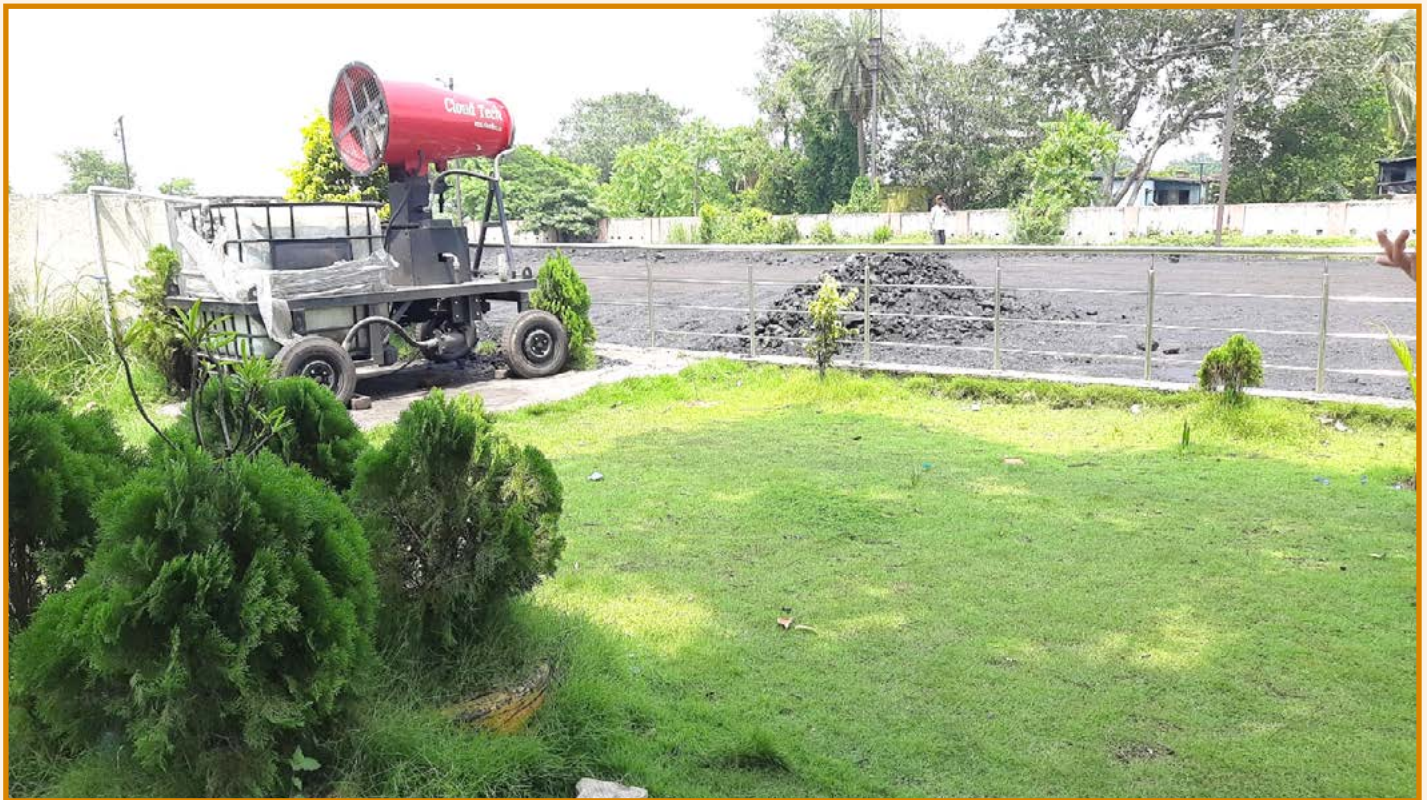
TROLLY MOUNTED FOG CANNON, BANKOLA RAILWAY SIDING
