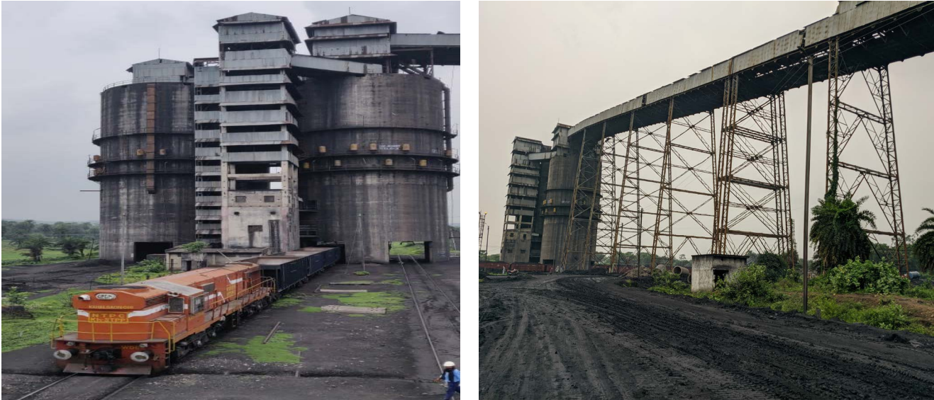
SILLO Loading at Rajmahal Area
