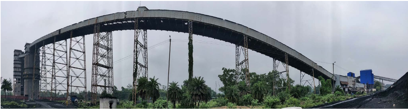
CHP at Rajmahal Area
