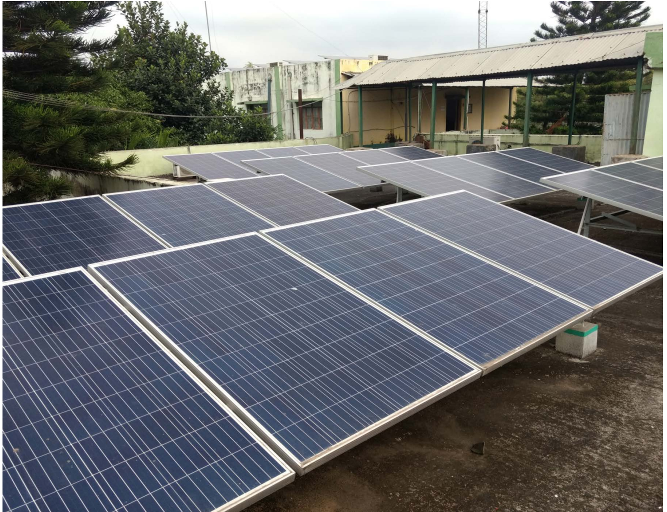
Installation of Roof-Top Solar Plant
